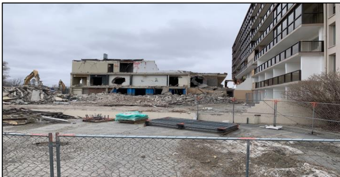
Progress during demolition, Rochelle
