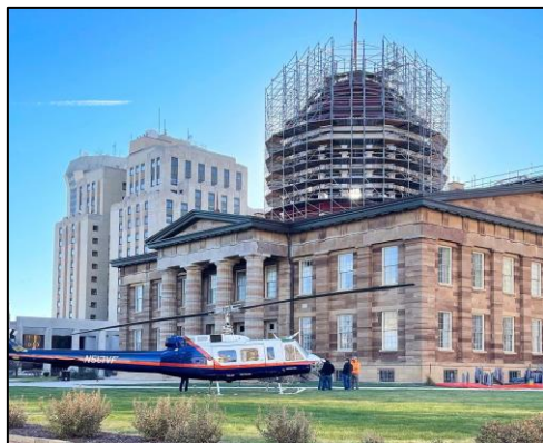
Old State Capitol Building flagpole removal
