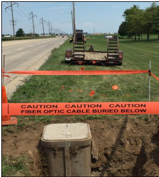
Decatur fiber project
