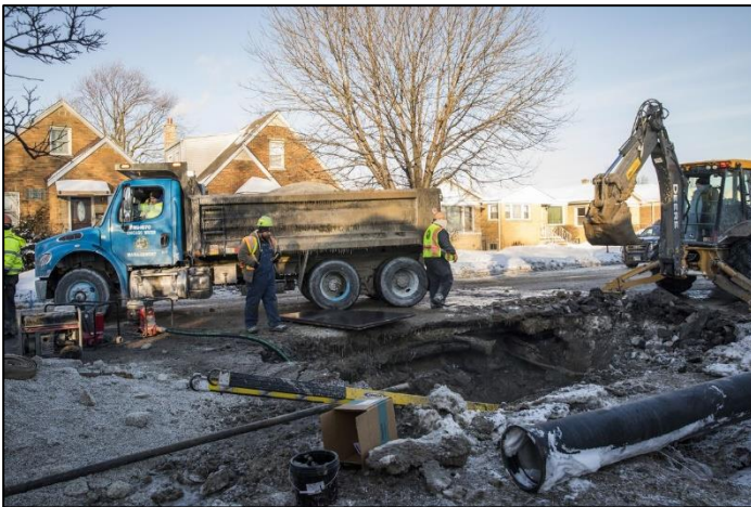
Lead service line replacement construction in Chicago
