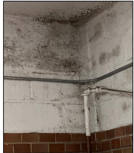
Mold in the Logan Correctional Center gym is being remediated by CDB.
