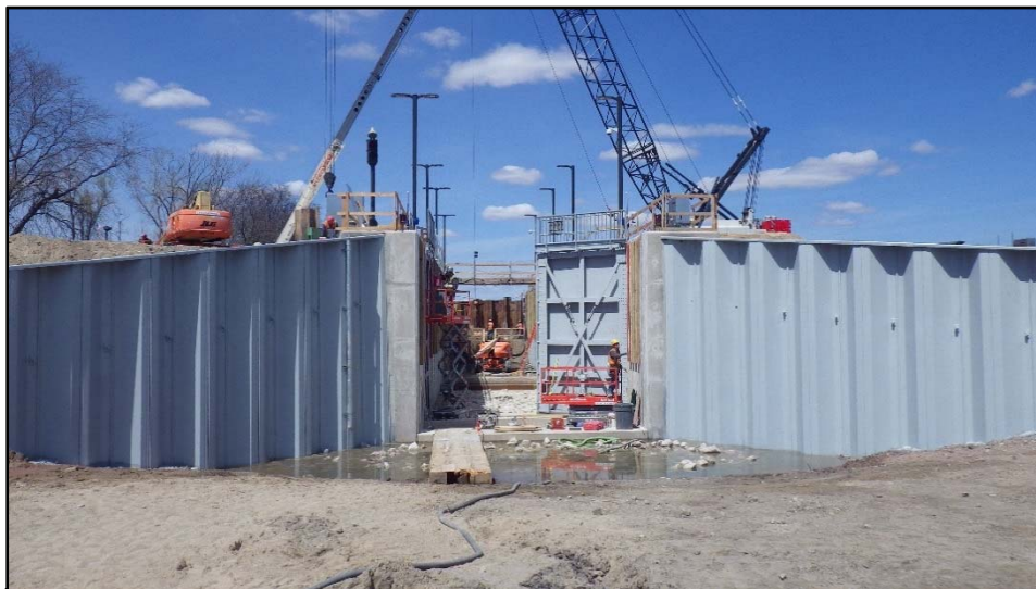
THE LOCK GATE DURING CONSTRUCTION AT THE STRATTON LOCK AND DAM
