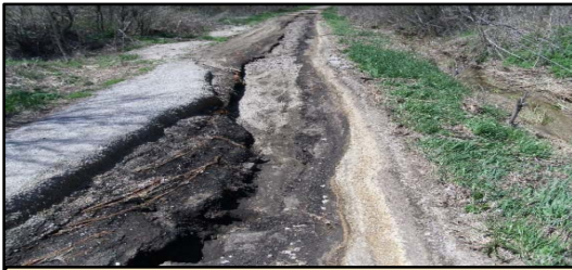
WATERWAYS HAVE FLOODED OUT PORTIONS OF ROCK ISLAND TRAIL AND ARE SLATED FOR RESTORATION USING FEDERAL FUNDS
