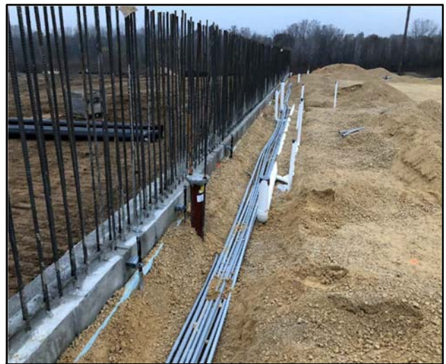
INSTALLATION OF ELECTRICAL CONDUIT AROUND THE PERIMETER OF THE TREATMENT BUILDING FOUNDATION AT THE SOUTHEAST ROCKFORD SUPERFUND SITE
