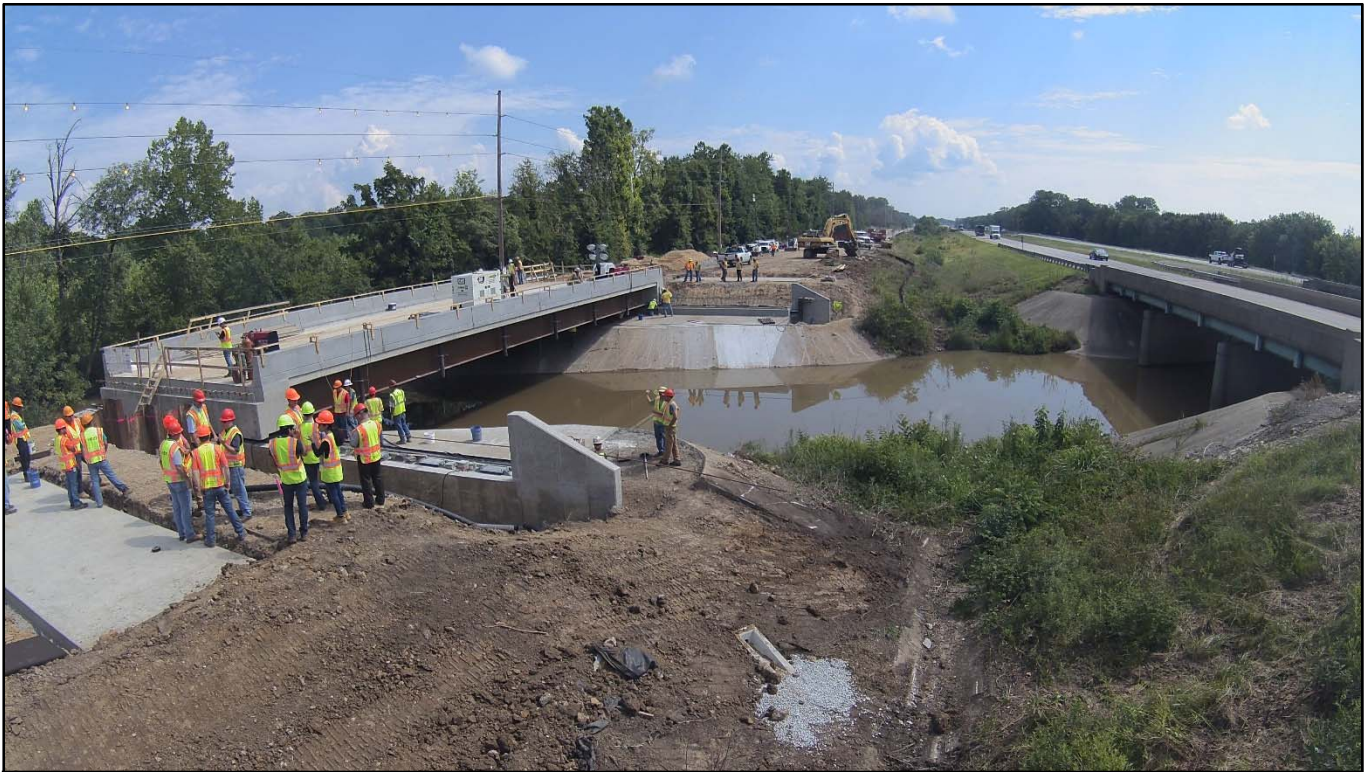
CONSTRUCTION OF A SLIDE-IN BRIDGE IN BOND COUNTY, IN 2017
