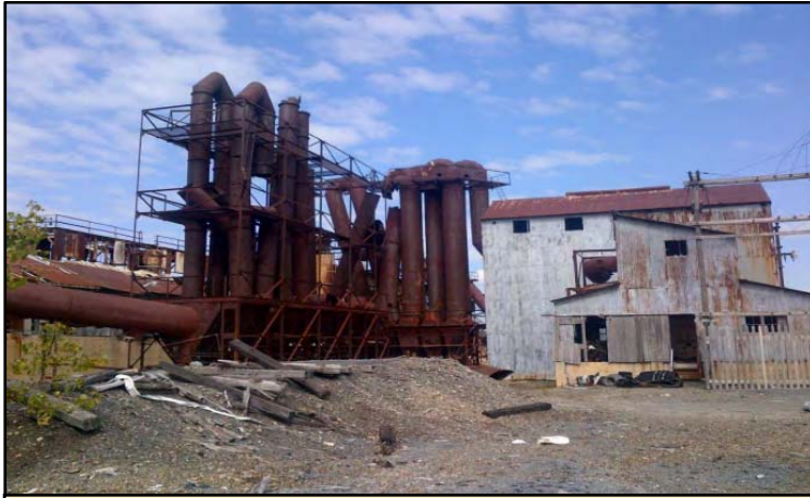
FURNACE ROOM AND COOLING TOWERS AT THE EAGLE ZINC SUPERFUND SITE
