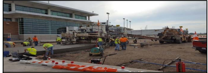
PEORIA AIRPORT CONSTRUCTION
