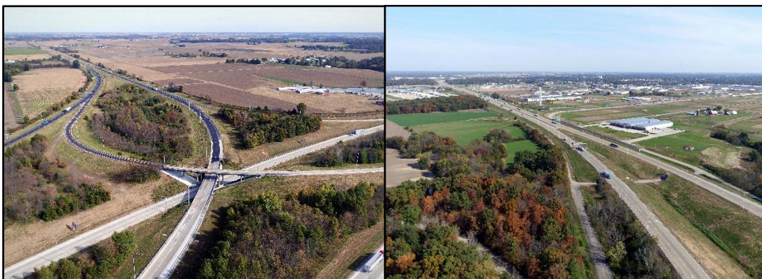
AERIAL VIEW OF THE I-57/70 RECONSTRUCTION PROJECT
